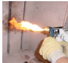
Ignition of the gun (over 3sec air cap could be damaged)
