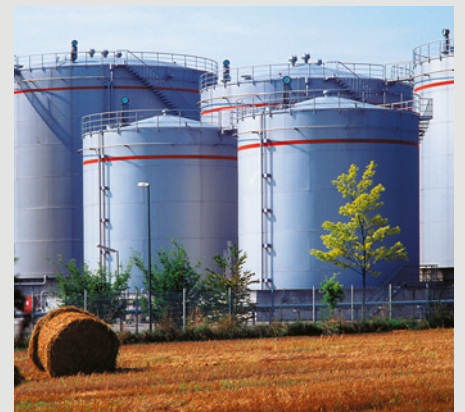
Industrial steel constructions
