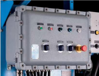
Pressure encapsulated housing
